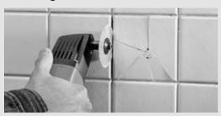
Use the diamond saw blade to cut out marble and concrete trass joints as well as to make grooves in plastered walls, dry wall, sheet rock, porous concrete.
